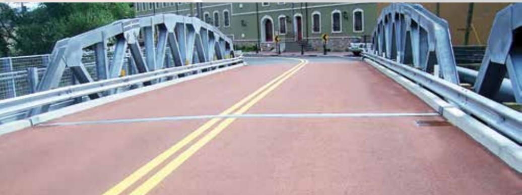
**APPLICATION** | High Friction Bridge Deck Overlay
