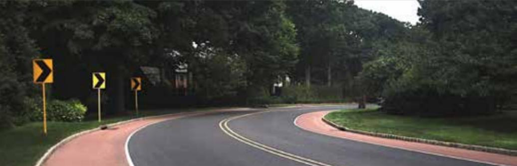
**APPLICATION** | High Friction Horizontal Curve Overlay
