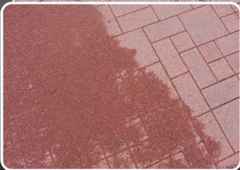
Kafka Granite Sunset Pink Granite Aggregate used at Buckingham Fountain in Chicago, IL.
